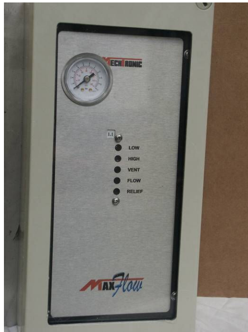
Figure 8 Typical view of special gas extractor control unit (mechanical)
