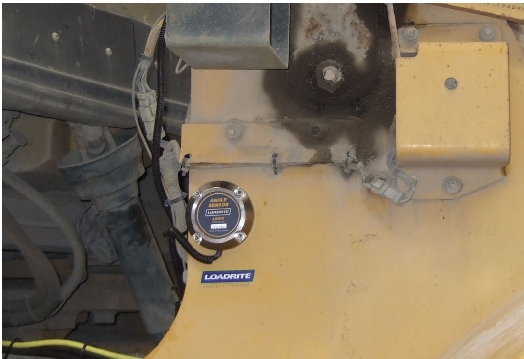
Figure 6 Typical LR966 inclinometer installation
